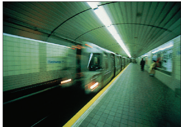
Tunnels are a common application.
