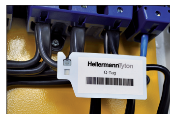
Q-tags can be labelled with pre-printed labels or by hand.
